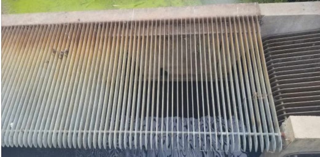
Figure 4. Photo of installed Ducks Unlimited barrier system from Lost Island Lake project in Iowa.
