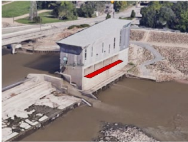
Figure 1. Southeast (downstream) view of the North Powerhouse, including proposed location of invasive carp deterrent.
