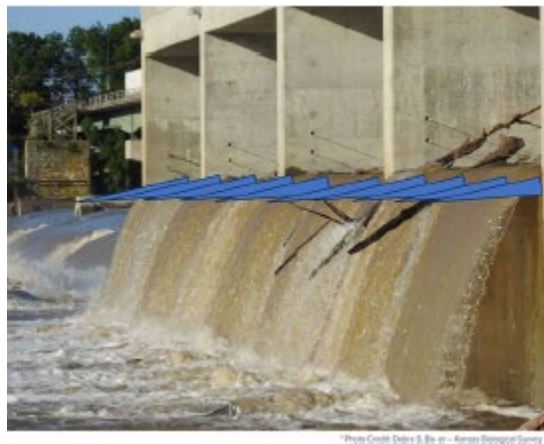
Figure 2. Concept sketch of the North Powerhouse, including the proposed location of the invasive carp deterrent.
