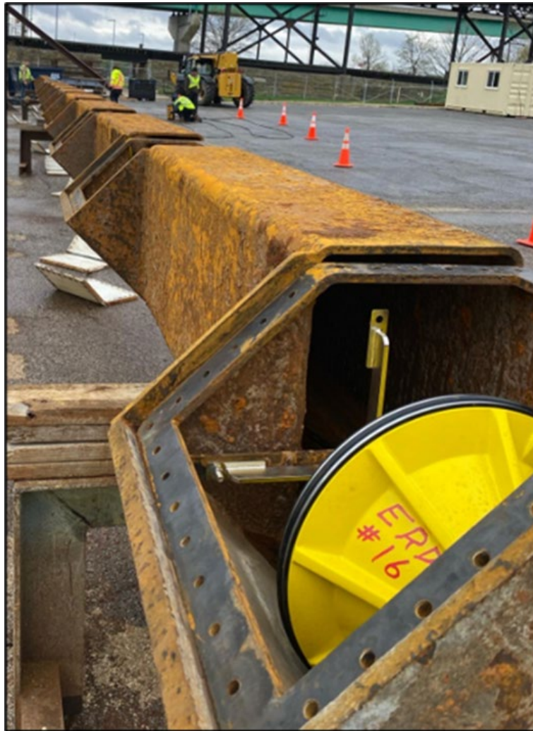
Figure 4. Updated speakers that are equipped with wet-connections to facilitate replacement underwater (Photograph by Marybeth Brey, USGS).
