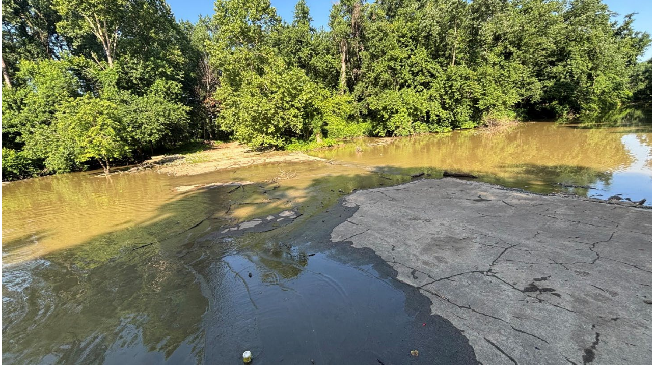
Figure 12. A photo of the Hovey Lake drain water control structure on June 23, 2025, when a river rise caused water to backflow over and through the structure into Hovey Lake. The river height at JT Myers L&D (USGS-03322420, Ohio River at Uniontown Dan, KY) was at 31.1 ft.
