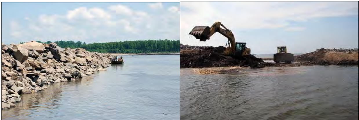
Figure 6. Dyke notching of 225 dykes has opened up additional habitat to aquatic life between river miles 212 and 953.5 on the Mississippi River. These efforts help ensure fish and other aquatic life are not stranded following high-water events when they seek flow refuges in the shelter of these structures. For some species they also provide spawning, feeding, hunting, and/or shelter habitat.
