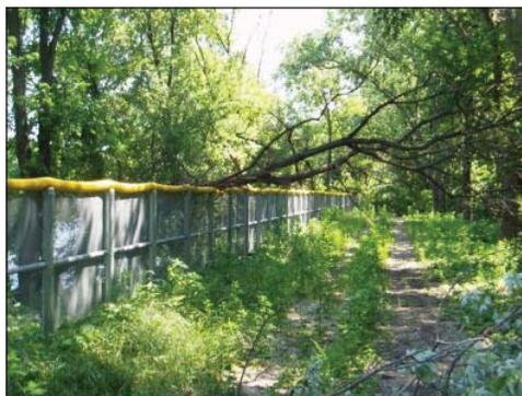
*View of a portion of the carp fence designed to prevent Asian carp movements into the CAWS from other waterways during periods of flooding. (Phil Moy Photo)*
