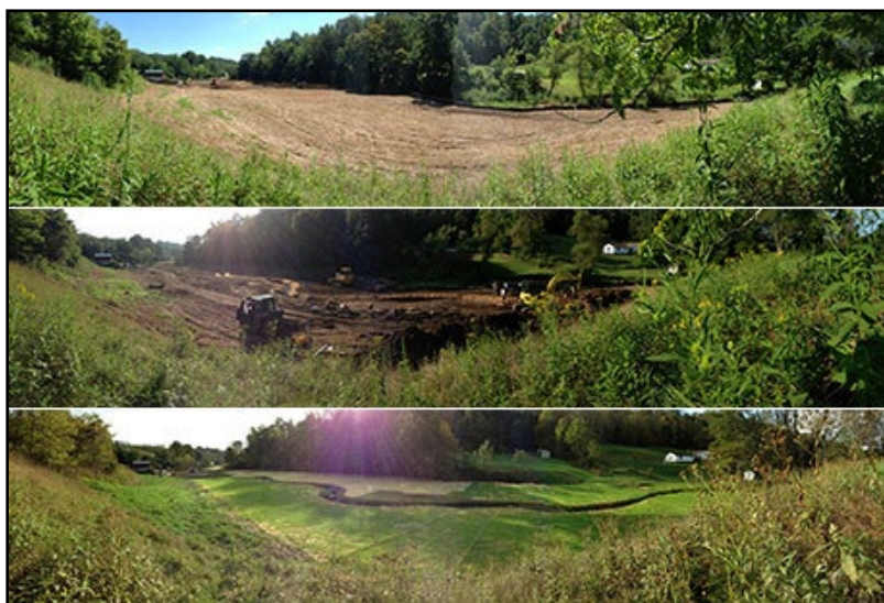
Before, during and after views of the Grave Creek mitigation site east of Cameron, WV developed as mitigation for a construction project. Resource Environmental Solutions, LLC Photo.
