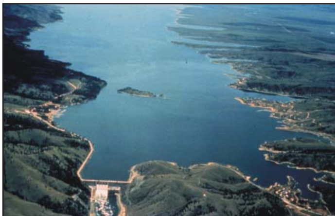
Gavins Point Dam and Reservoir, SD.
